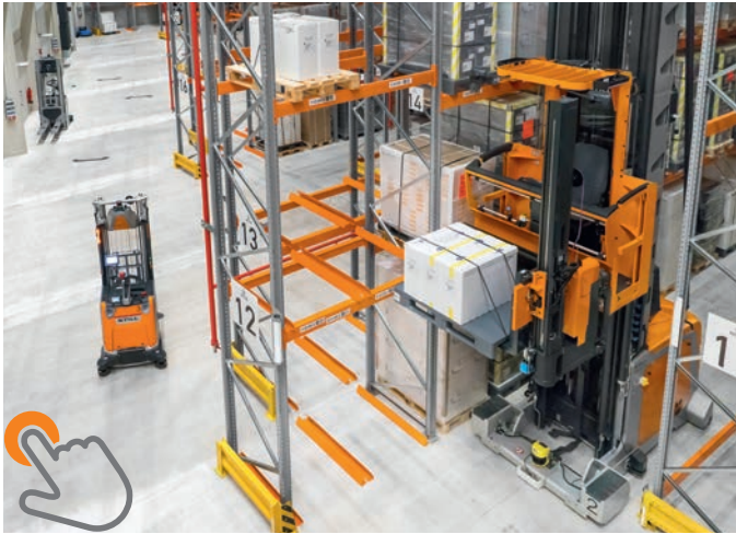
Customised and flexible: An automated materials warehouse for Vetter
